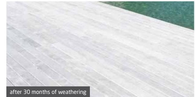
This deck in Oesingen was photographed when newly installed (left), after 10 months (middle) and after 30 months of weathering (right).
